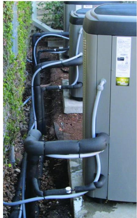
All three systems communicate via the Lennox I-Comfort WiFi controllers, one in each zone. Shielded control wire ensures reliable communication.
